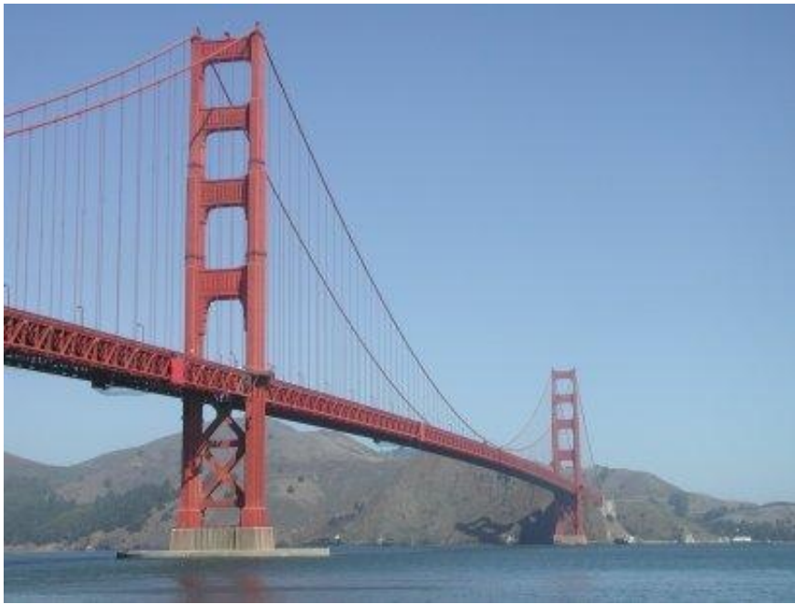
Golden Gate Bridge, San Francisco
